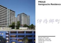
Site area: 2,640,71 sqm Building area: 1,089,53 sqm Total floor area: 8,749,42 sqm Structure: RC Floors: 13 abovegrout 1 underground Height: GL+40.02 m Units 98 units
