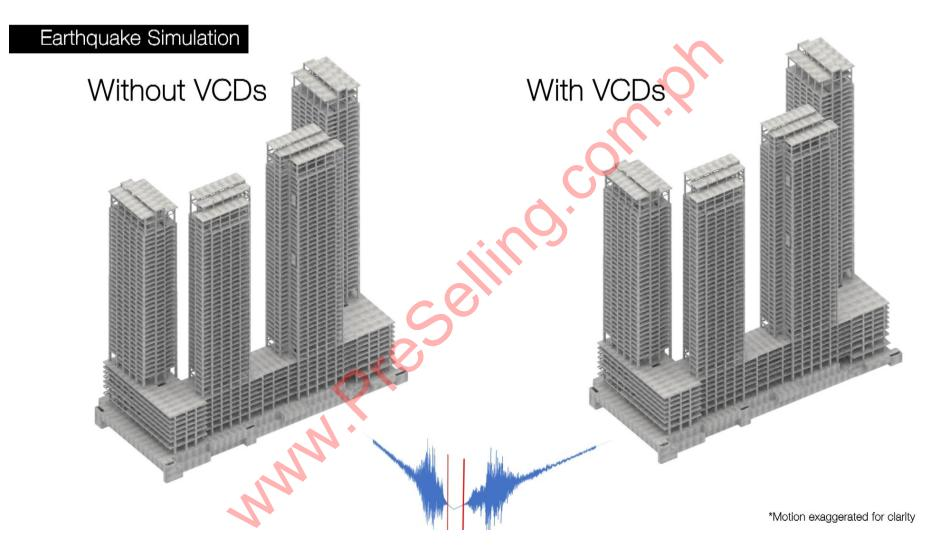
Animation shows a sample comparison of Big Apple development subject to a far-field earthquake from the Manila Trench comparing damped structure with VCDs to low-inherent damping structure without VCDs.
